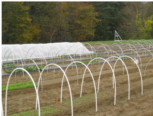
Low tunnel bows constructed of PVC (front) and EMT (back).
