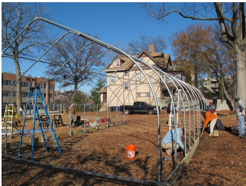
Photograph: Construction of a 20 by 36 feet high tunnel (EastPoint, Rimol Greenhouse Systems, Inc.) in East Orange, NJ.
